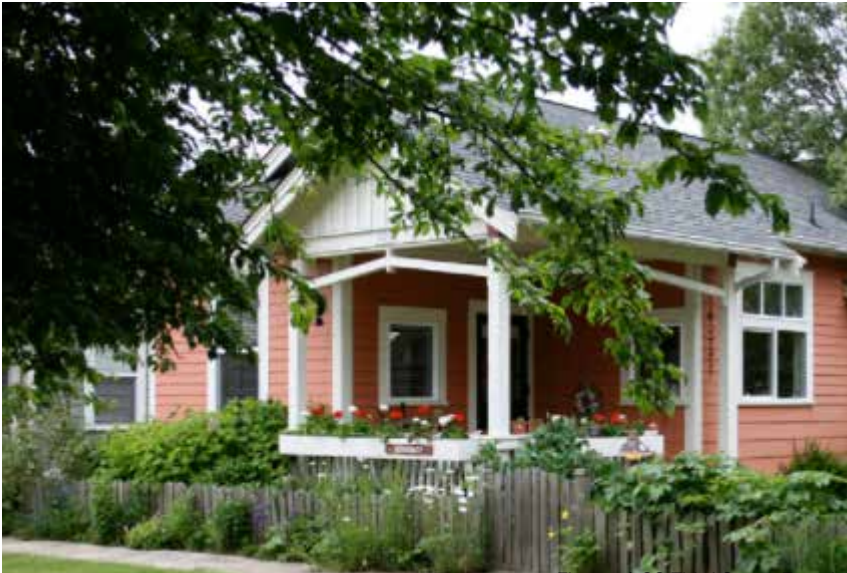
Figure 1.33 Third Street Facade
